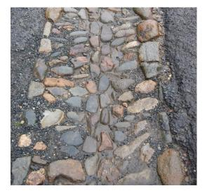
Pull / lever out loose cobbles and cobbles riding more than 20mm higher or 20mm lower than adjacent cobbles.
